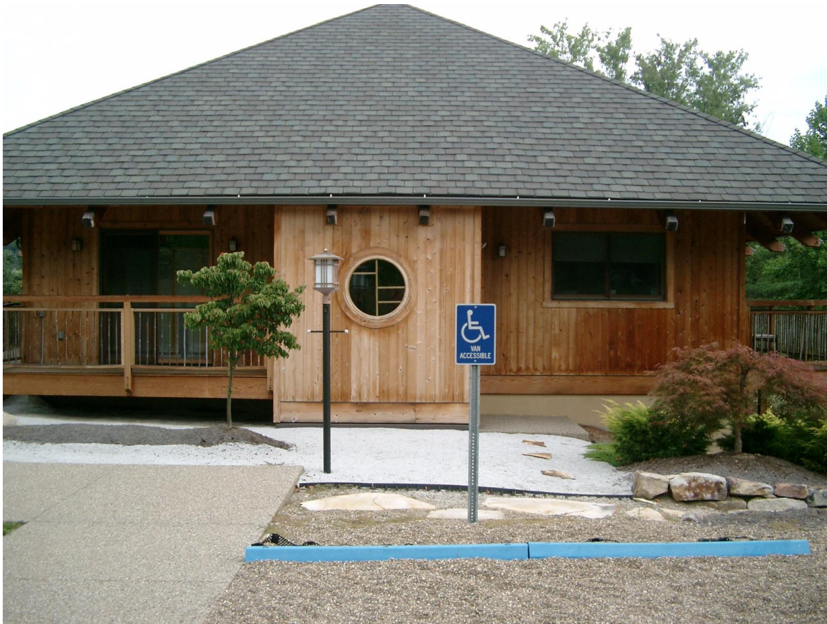
Front View of Changing Signs Learning Center Building
