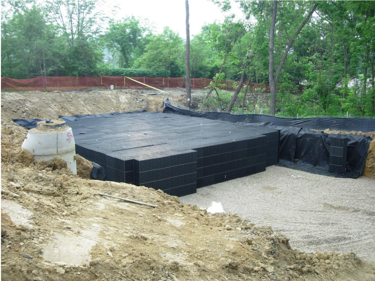
Lakeview Square Rain Tank - During Construction
